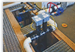
Nursing Home, OH 2 Salcor 3G UV Units in Series with an Activated Sludge Plant. Replaces Chlorination
