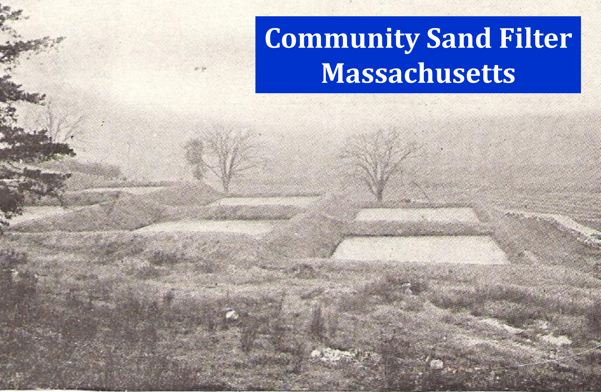
FIG. 37.—View of Sand-filter Beds for Village in Massachusetts.
