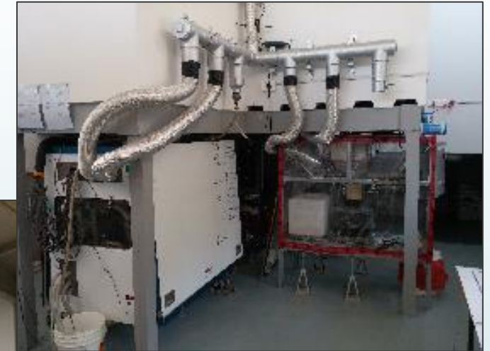
Engineering prototype installation in India in mid-2017.
