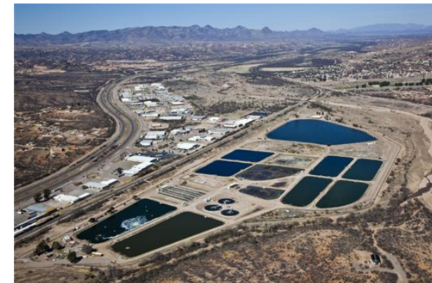
Nogales International Wastewater Treatment Plant
