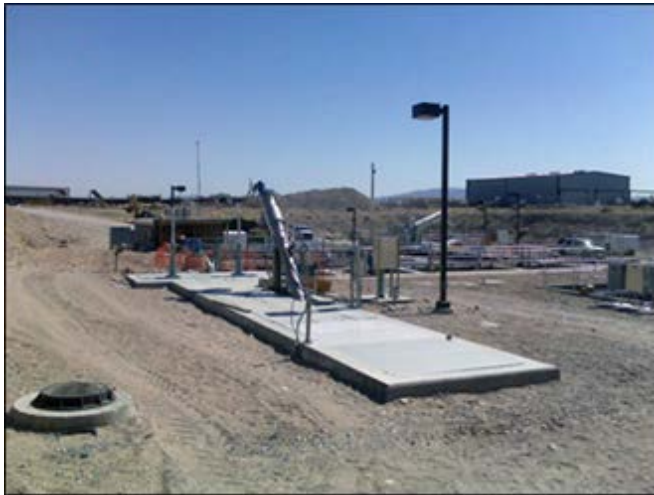
EPCOR Wishing Well WWTP, Ft Mohave, 1 mgd, Valentine Engineering photo
