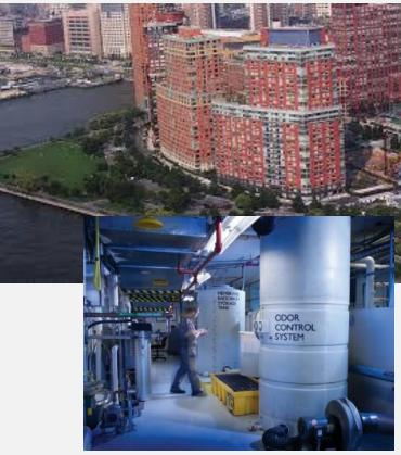
25,000 gpd of wastewater Membrane Bioreactor Toilet Flushing, cooling, irrigation
