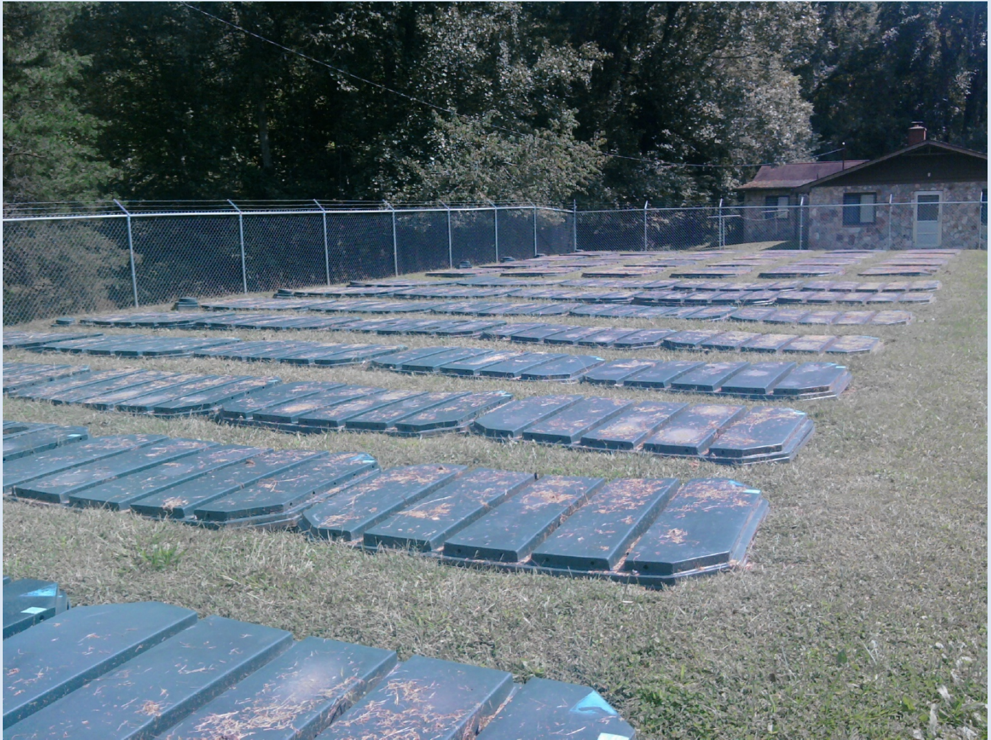
Field of Peat Fiber Module Filters
