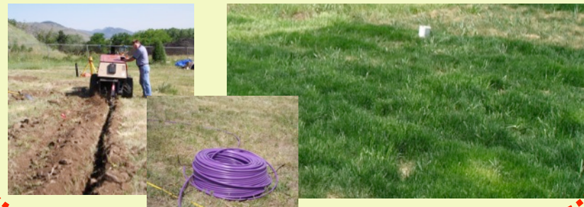
Shallow subsurface drip dispersal for turf irrigation
